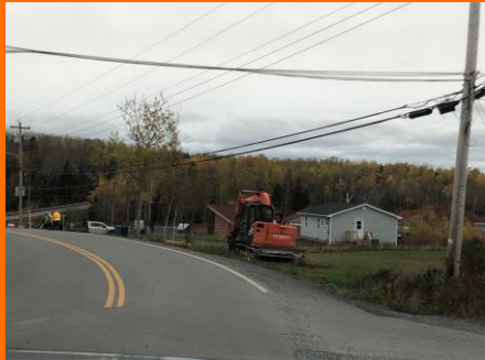
New Sidewalk is coming along nicely in the community.
