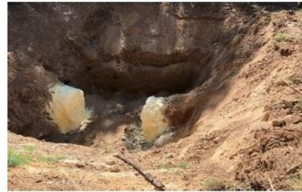
Original Piece of pipe removed in September 2020
